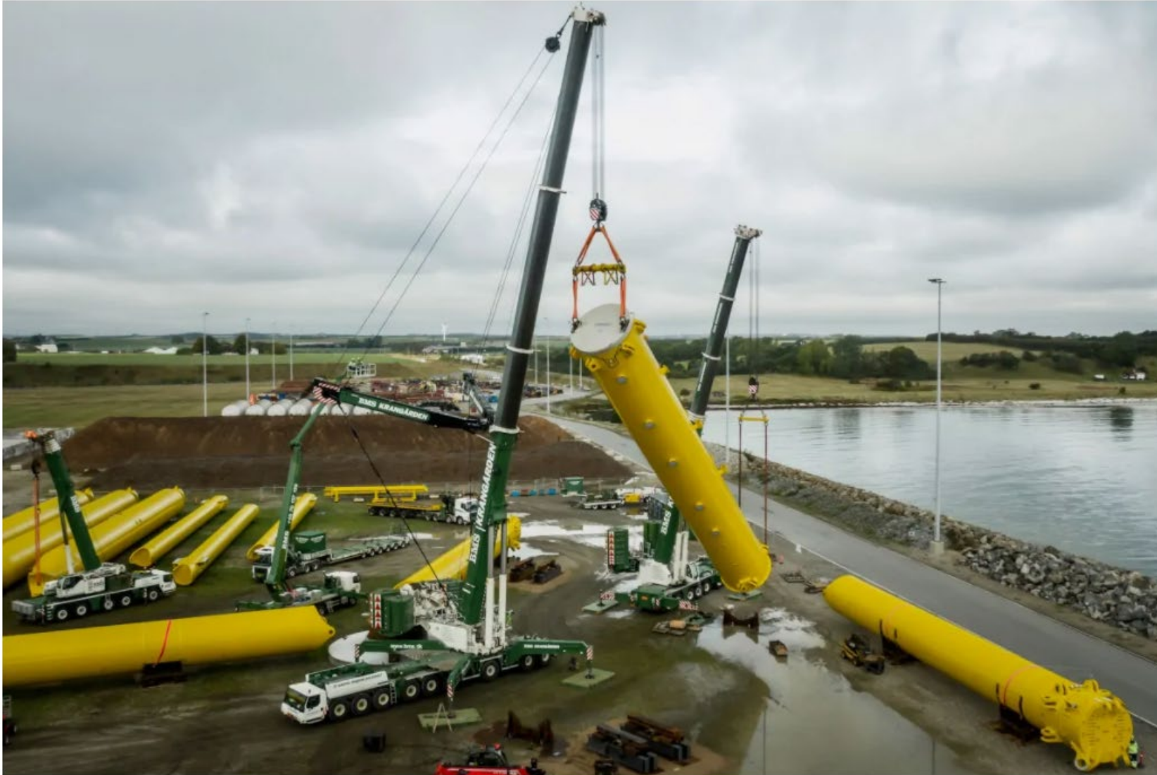
Up-ending of the center column at the port of Grenaa, Denmark. Photo credit: The TetraSpar Demonstrator Project ApS
