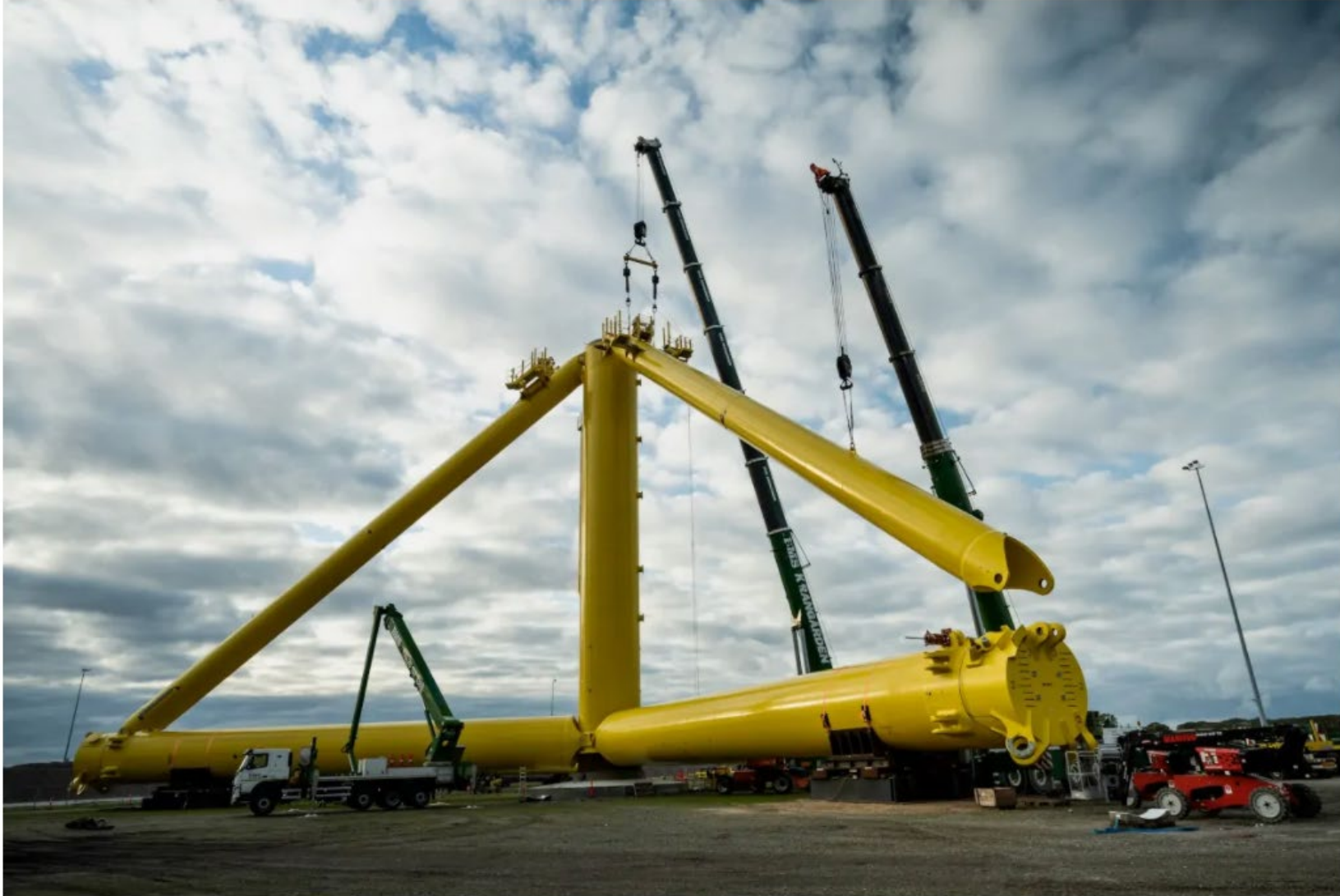
Mounting of the diagonals using maintenance-free proprietary technologies for fast assembly. Photo credit: The TetraSpar Demonstrator Project ApS
