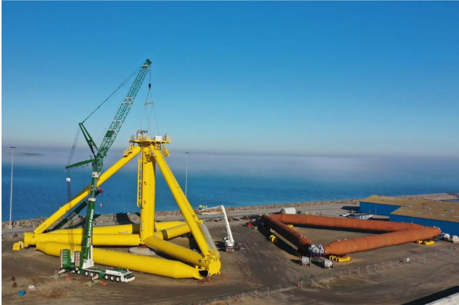
Completed foundation and keel. Photo credit: The TetraSpar Demonstrator Project ApS
