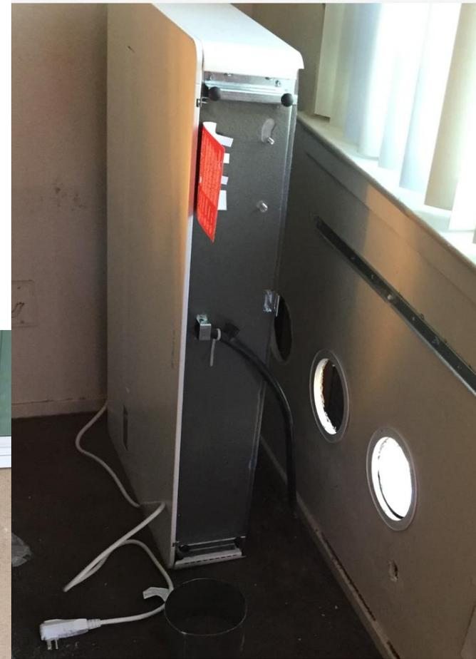
First US installation of 120V HPs – avoids panel upgrades and asbestos mitigation costs
