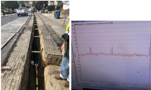
Pilot deployment and Strain Test Signal at a DIMP Fault Crossing Site
