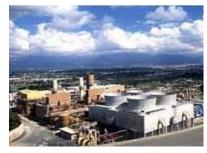
The Puente Hills Landfill Gas-to-Energy facility is a 46 MW conventional Rankine Cycle Steam Power Plant that uses landfill gas (LFG) as fuel to generate electricity. LFG is fired in the plant's boilers producing superheated steam. The superheated steam is used to drive the steam turbine/generator to generate electric power. The Puente Hills Landfill Gas to Energy facility was constructed by Los Angeles County Sanitation District and began full commercial operation in January 1987 and has
