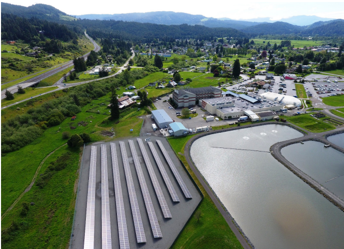
In 2017, the Blue Lake Rancheria completed an award-winning microgrid project that includes a 420-kilowatt solar array and nearly 1 megawatt-hour of energy storage. The system can automatically disconnect from the grid when needed to continue powering critical infrastructure, preparing the local community for the impacts of wildfires, earthquakes, and tsunamis.
