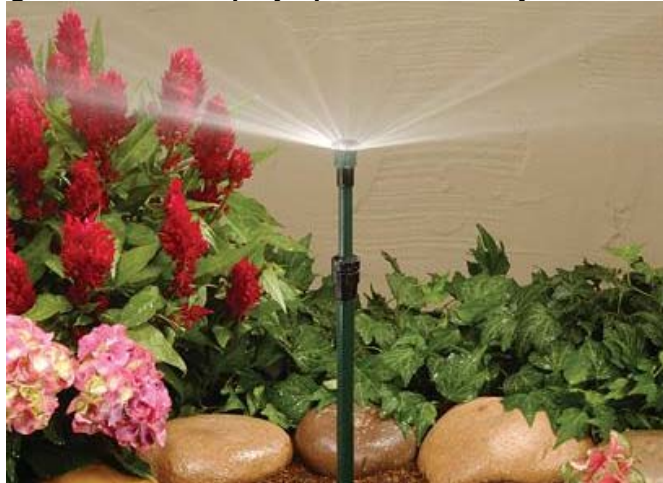
Figure 4-5: Shrub Spray Sprinkler With Adjustable Riser
