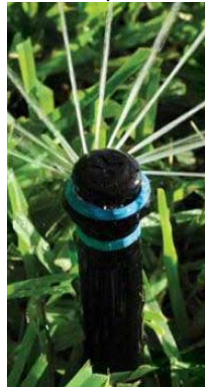
Figure 4-3: Pop-Up Multistream, Multitrajectory Spray Sprinkler
