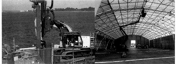
Preparing for Major Civil Works Installation of coffer dam at discharge canal and tents to manage wet canal sediment
