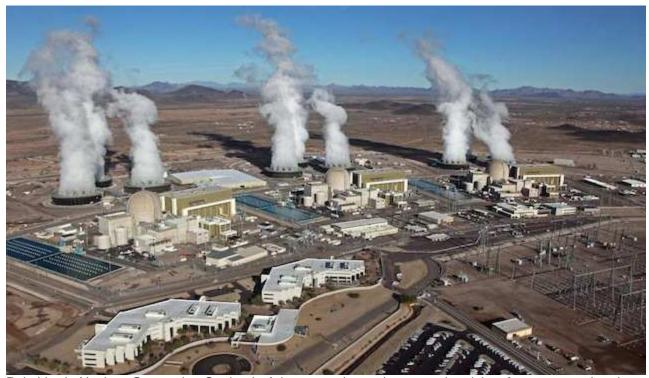
Palo Verde Nuclear Generating Station in Arizona produces the most electricity of any power plant in America, over 30 billion kWhs per year. In 2014, it ran almost 24-7, with a capacity factor of 98% (cf = energy actually produced divided by the maximum possible). No other energy source but nuclear approaches a cf of 90%, and most are under 50%. Source: NEI
