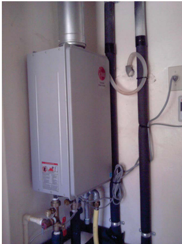
Figure L.1. Tankless hot water heater unit
