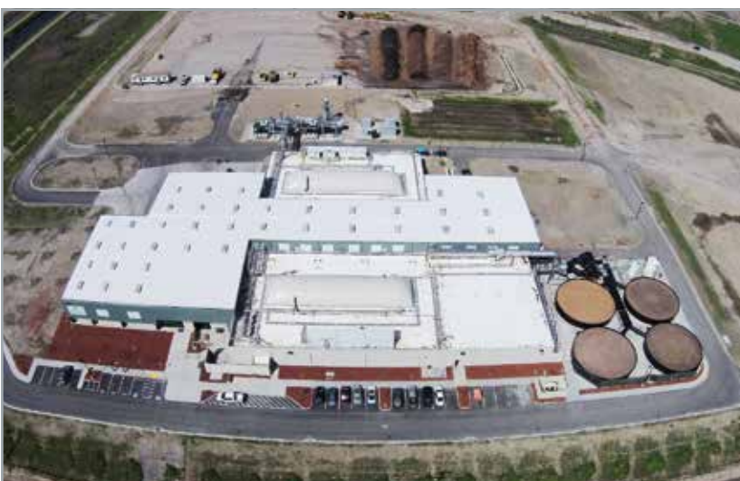
San Jose's facility can convert 90,000 tons of waste to 1.6 MW of renewable electricity. The facility was developed by Zero Waste Energy Development Company and is part of the city's zero waste by 2022 plan.
