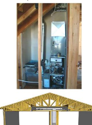
Figure 6: Interior Furnace with Ducts in Conditioned Plenum Space (IBACOS 2013)
