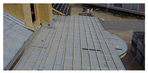
Figure 9: Ventilation for Tile Roofing – Counter Batten (CBIA Forum)
