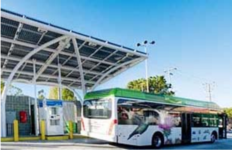
Emeryville: co-located car and bus fueling; H 2 from solar electrolysis and liquid delivery
