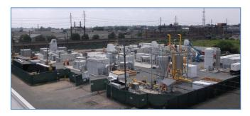
In May 2013, energy company **Dominion**, broke ground on a 14.9-MW fuel cell power – generating facility in Bridgeport, Connecticut – enough electricity to power approximately 15,000 homes. FuelCell Energy will build, operate, and maintain the facility, which will include five Direct FuelCell<sup>®</sup> stationary fuel cell systems and an organic rankine turbine that will
