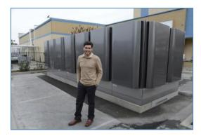
Asian food product manufacturer, Ramar Foods International, has installed a 200-kW Bloom Energy fuel cell at its Pittsburg, California, manufacturing and packaging plant. The fuel cell system will provide 65 percent of the site's electricity – which will save the company at least \$15,000 each month – and will reduce the plant's carbon footprint of by over 400,000 pounds annually.
