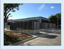
**Honda** installed five Bloom Energy fuel cell systems (totaling 1 MW) to provide 25 percent of the electricity needs for its 1.13 million square feet (sq. ft.) of office space, research, design and development operations, and parts distribution center in Torrance, California. The fuel cells, which run on natural gas, will reduce Honda's carbon dioxide emissions by approximately 16 million pounds over 10 years.
