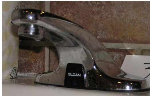
Sensor-operated Faucet – handicap stall
