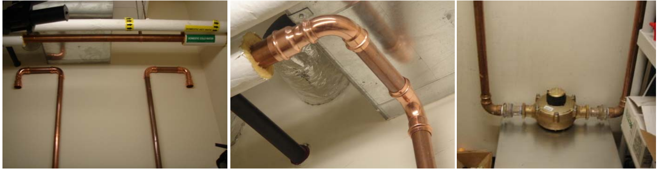
The above photographs show existing supply piping, piping modifications, and the new water meter.
