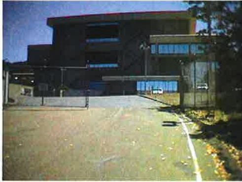
Power Plant Entrance
