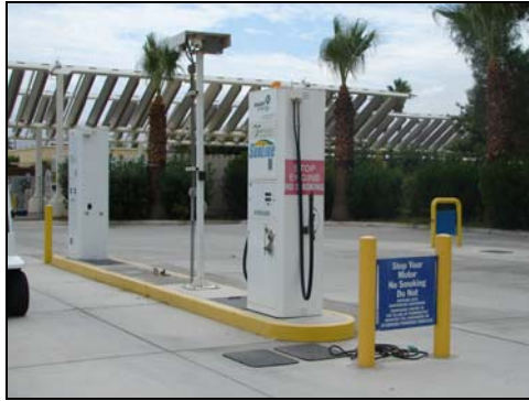
Figure B. SunLine Transit fueling station
