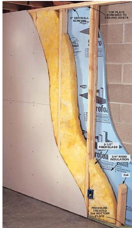
Figure 0-21 – Brick wall with furring details
