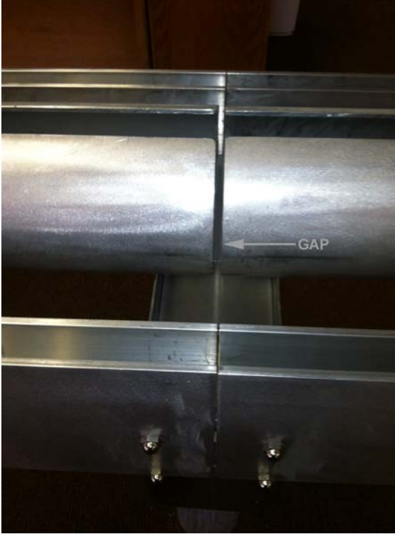
Figure 3d - Vehicles traversing the guideway can pass over gaps without any contact. Gaps also allow for thermal expansion of rails without warping or buckling common in rail systems.
