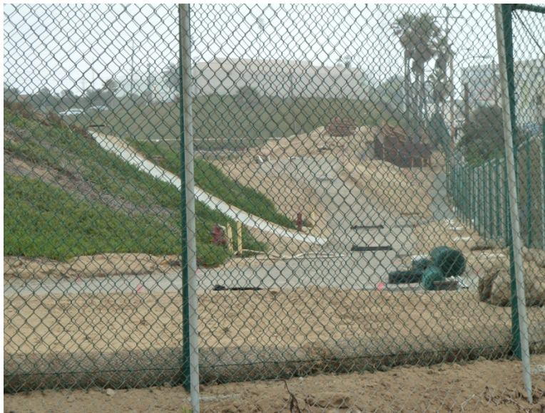
Figure 5a: Asphalt road leading to new berm and side view of concrete spillway.
