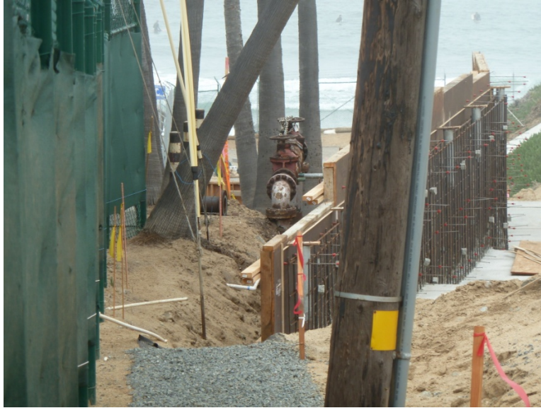
Figure 2a: View of concrete retaining wall under construction on July 11, 2012. The existing palm trees and backflow preventer can be seen in this view.
