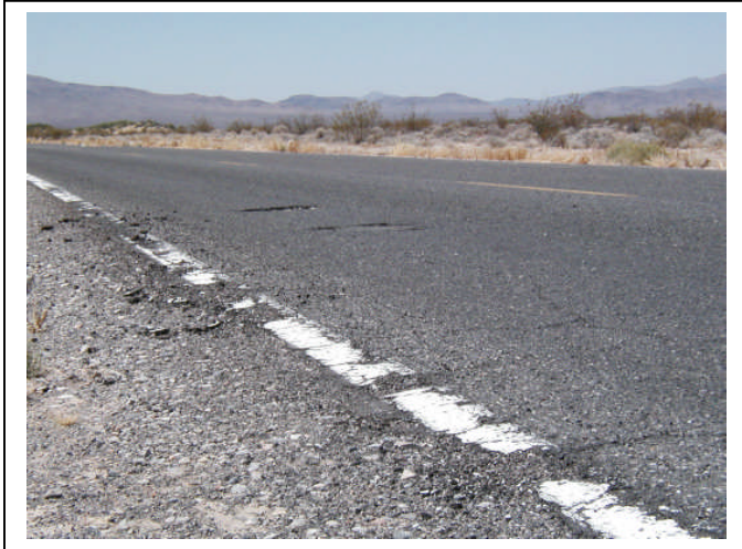
Potholes and crumbling curbs located on the “Nevada” side of Old Spanish Trail Highway looking Southwest about 3-4 miles from the proposed project site. 5/17/12
