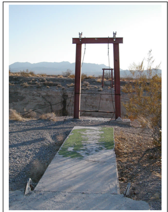
What's left of the bridge....12/20/11
