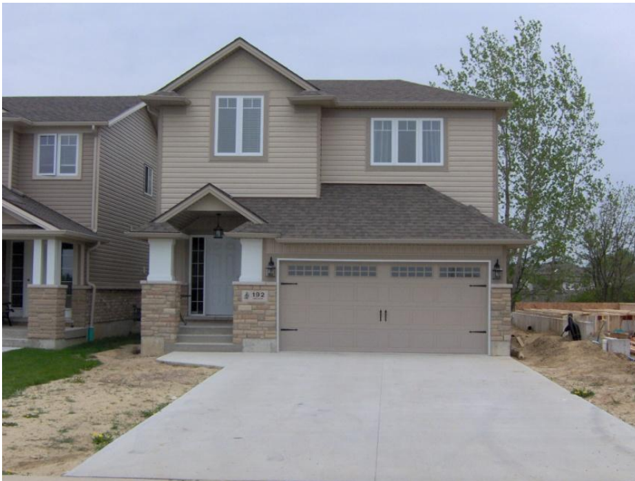
New Construction – 2-storey plus finished basement
