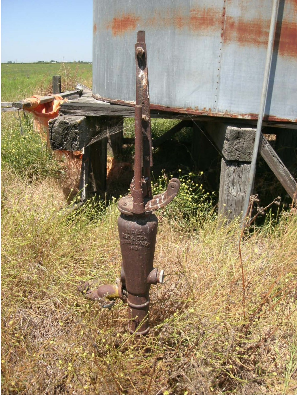
Photo 4. View of water pump facing north.
