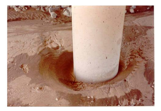
Figure 5. Local scour around bridge pier
