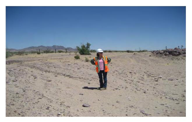
Figure 17. View toward southeast of channel downstream of bridge 709.4. This channel has been enlarged by excavation. It gradually vanishes to from sheet flow after about 1,000 feet.
