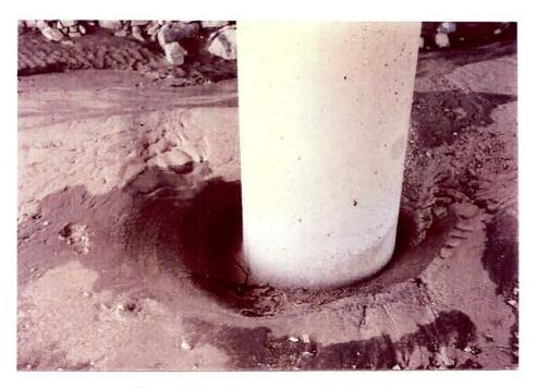
Figure 9. Local scour around bridge pier
