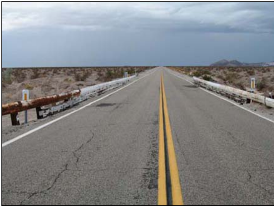
Typical Existing Above Grade View of NTH/Route 66 Bridge
