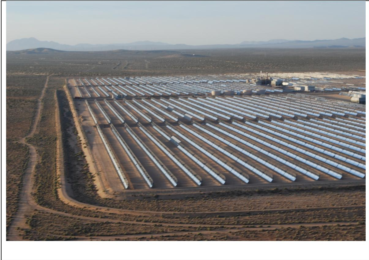
**Figure 4-2. A picture showing a parabolic mirror solar array at the Kramer Junction SEGS plant**
