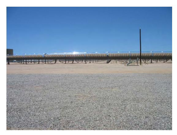
In this photograph, the mirrors are pointed vertically. The most intense reflection is from a joint connector on the normal to the observer. Reflections off the individual joints in the HCE tube are visible. Note the limited extent of glow and lack of reflection from the operating HCE tube visible on either side of the normal.
