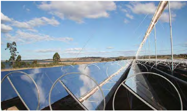
Linear Fresnel technology (Wikipedia.org, Fresnel_reflectors_ausra.jpg)
