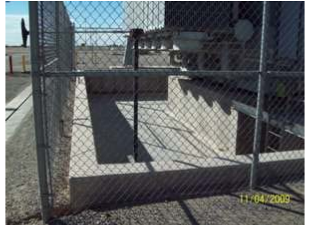
d. Transformer 11 (CTG 1) NE corner looking south, showing oil containment moat.
