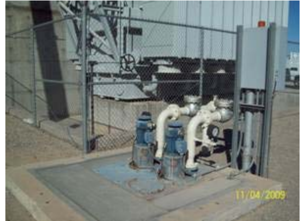
b. Transformer 12 (CTG 2) looking NW at SE corner. Rain water sump pump.
