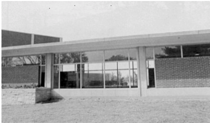
FIG. 3. Clear glass windows of a corridor showing see-through effect.
