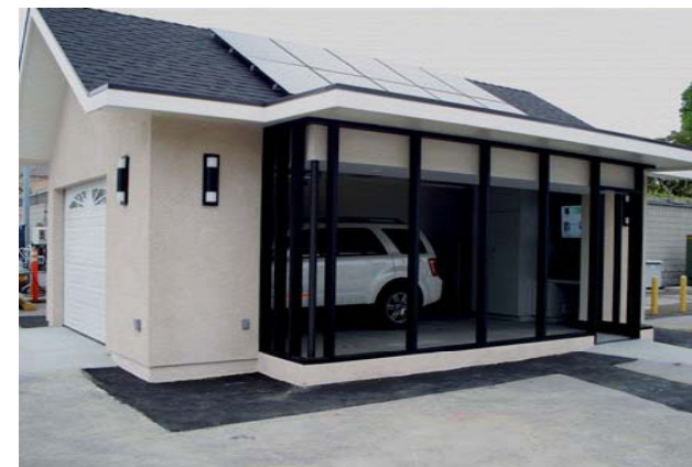
SCE's Garage of The Future is generating data related to the convergence of solar, stationary storage, vehicle charging and discharging and home energy management
