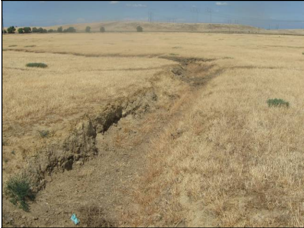
DRAINAGE (2A) Looking east at earthen channel
