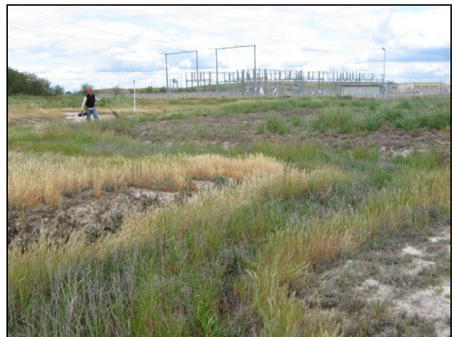
DRAINAGE WETLAND (D-2) Looking east from Bruns Road
