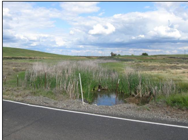
DRAINAGE WETLAND (D-4) Looking east from Bruns Road (30-inch-diameter cmp under road)
