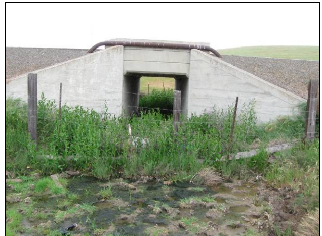
DRAINAGE WETLAND (D-1) Looking west; 6-foot by 6-foot box culvert under Bruns Road
