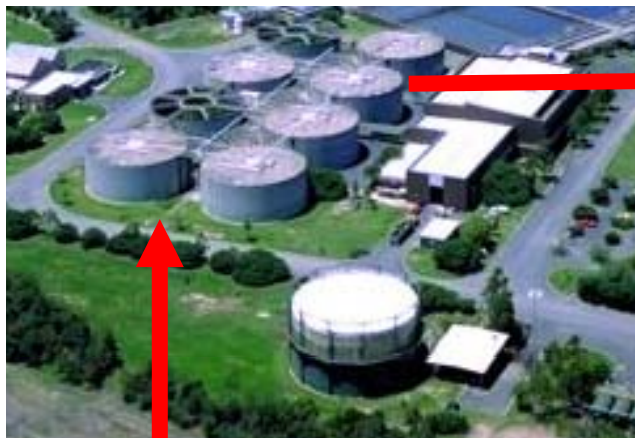
Wastewater or Dedicated Digesters
