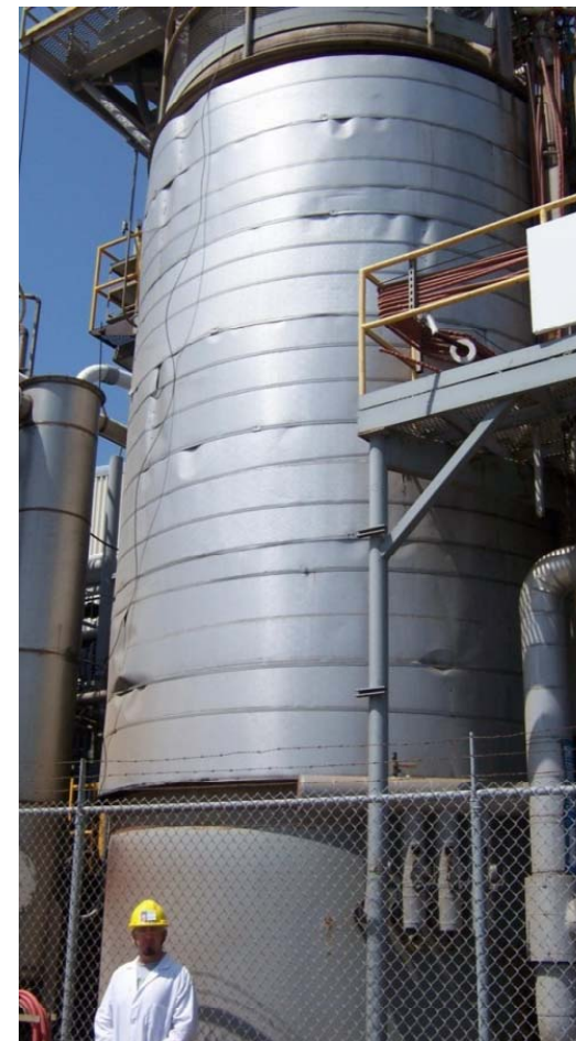
California fermentation facility
