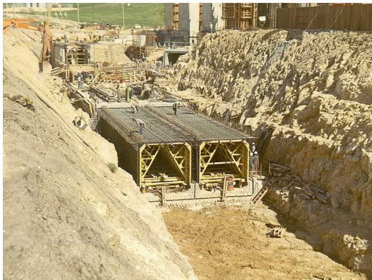
Figure 11 – Original Circulating Water Tunnel Excavation & Construction
