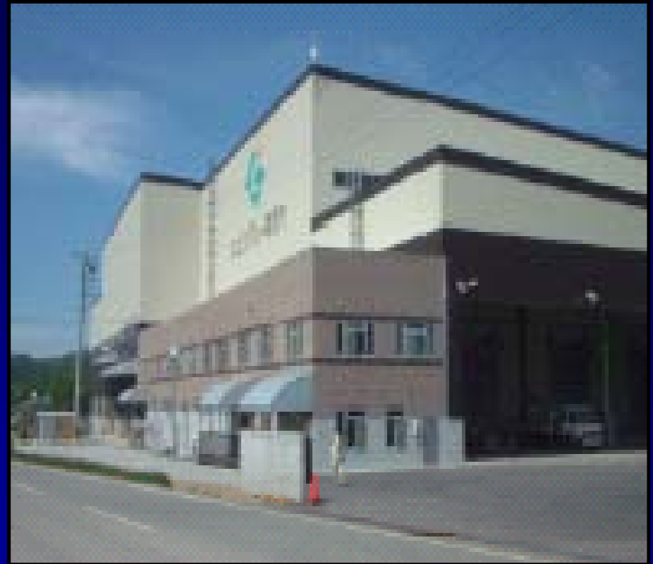
The Plasma Direct Melting Reactor (PDMR) at Utashinai, Japan converts unprocessed MSW and ASR to electricity, sand-size aggregate, and mixed metal nodules
