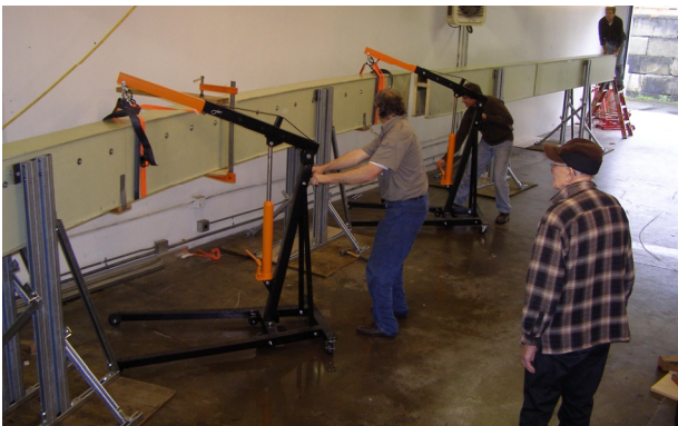
U.S. DOT Research & Innovation program maglev guideway installation.
