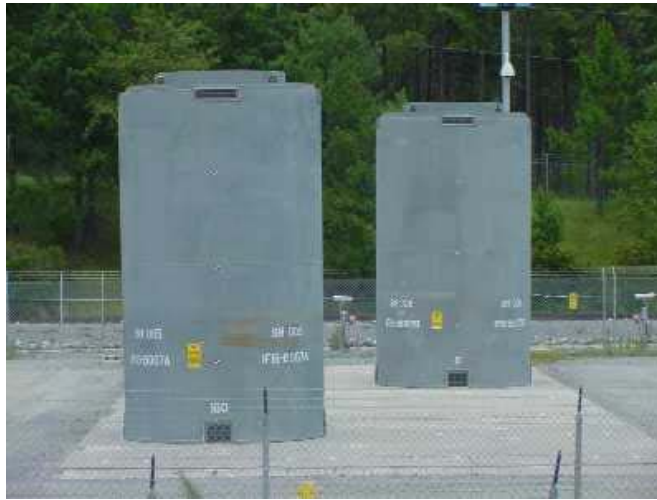
Figure 28: Photo of Loaded HI-Storm Casks at Plant Hatch 342
