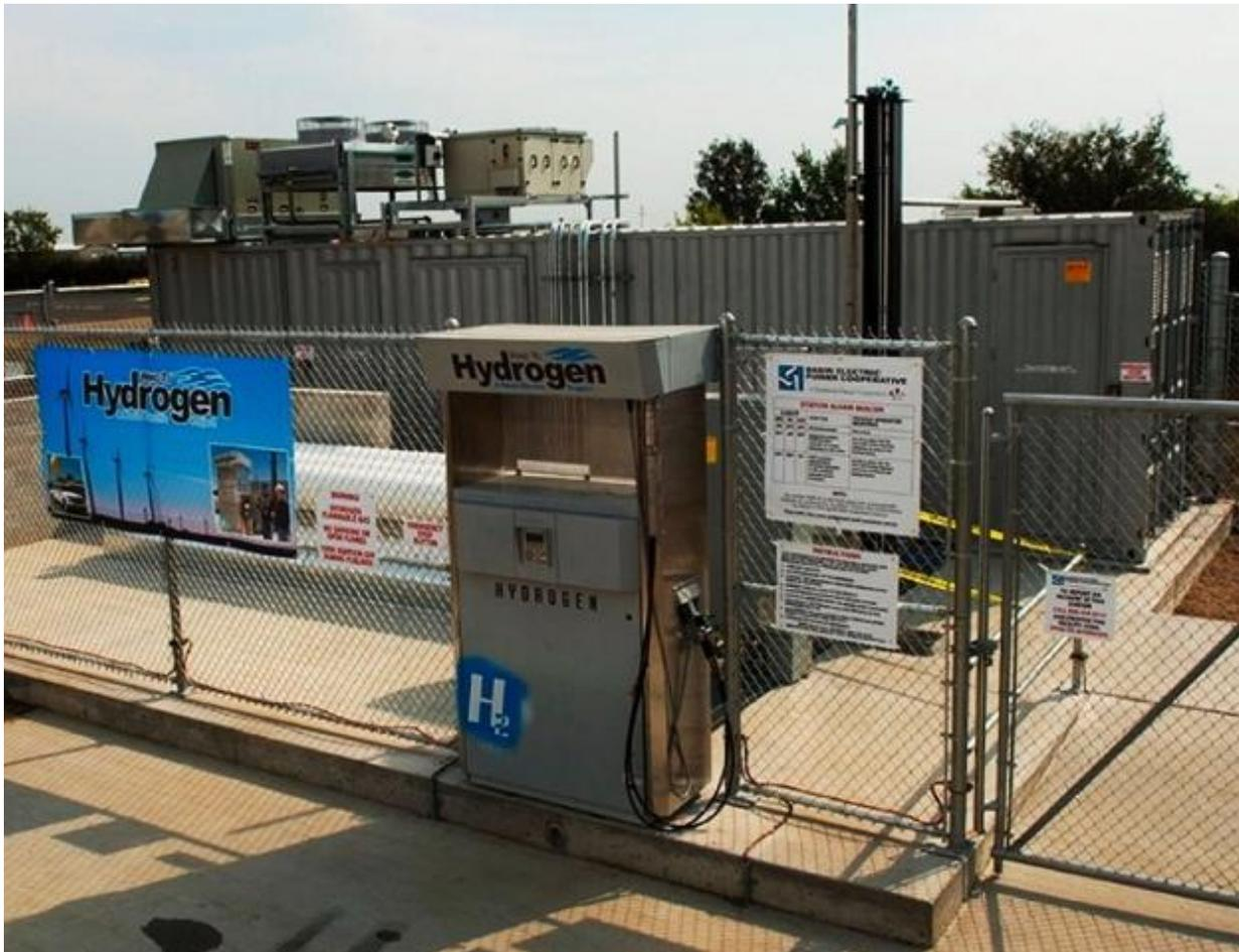
*Figure 2 – The electrolyzer system in North Dakota to be used for the first HYDRNOL demonstration.*
