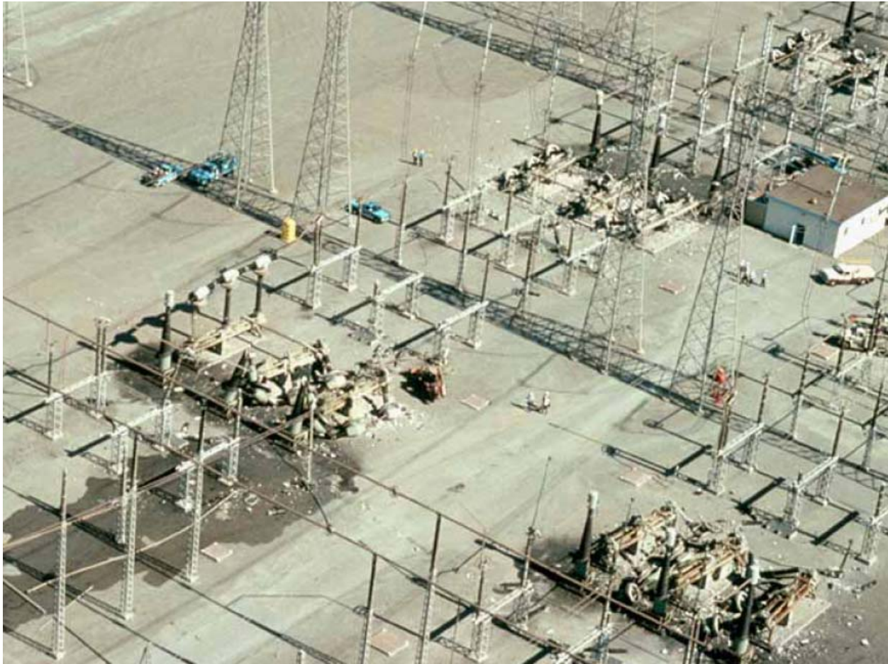
Figure 21: Moss Landing Switchyard after the Loma Prieta Earthquake, 1989 267
