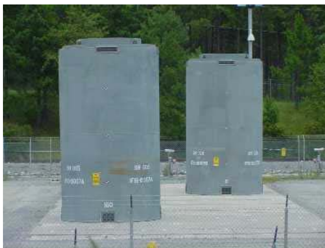
Figure 28: Photo of Loaded HI-Storm Casks at Plant Hatch 332
