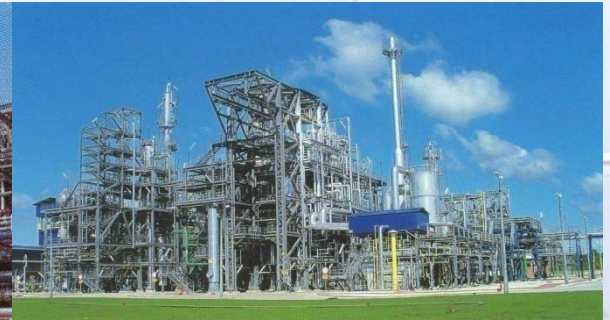
c) Molten Salt system with an output of 7.7 MW at 470°C, melamine plant in Germany
