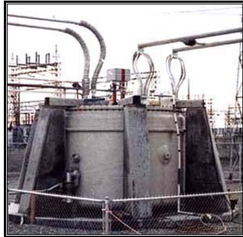
10 MW – 3 Sec. Coil Tested For Transmission Stability
