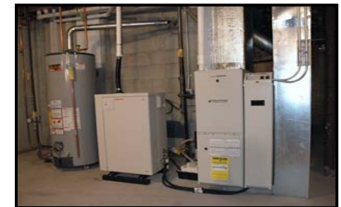
1 kW micro-CHP system for homes
