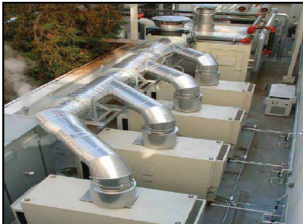
240 kW Micro-turbines / 100 T chiller
