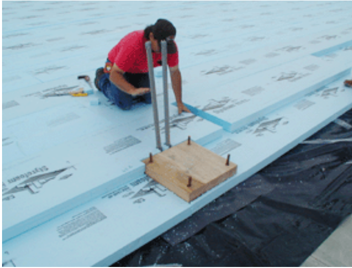
Freezer Floor Insulation
