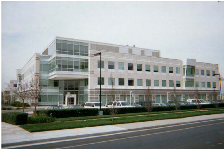
Figure 100. Site #1 – Office Building in San Jose
