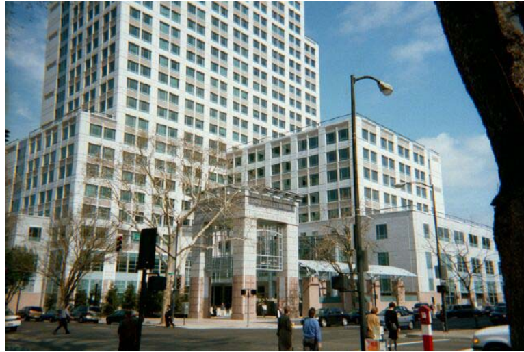
Figure 106. Site #3 – Southwest Corner View (Main Entrance)
