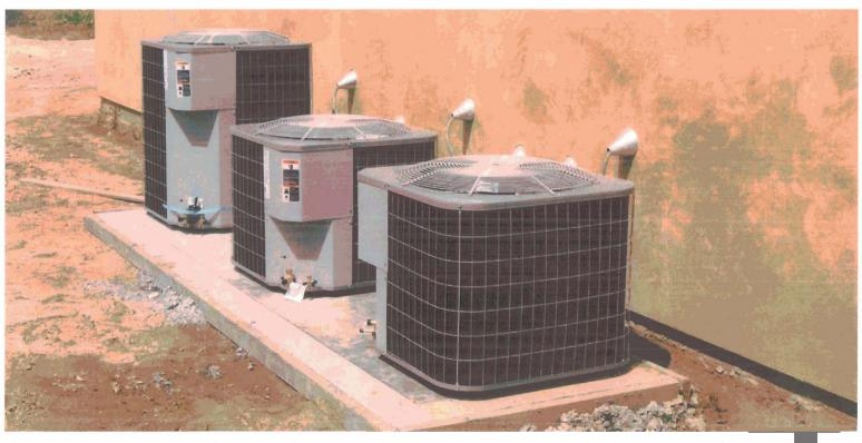
June 15, 2007 Bruce Wilcox ^ 9.5 Tons on a Fresno house ~ 10 KW compressor
