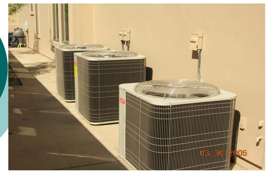
13 tons AC on a 3763 ft2 Palm Springs house 282 ft2/ton - 2.2 kW furnace fans
