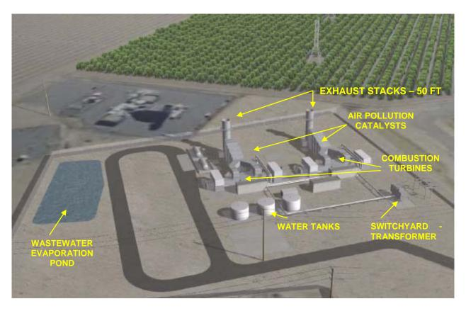
Air emissions from the proposed SPP would be controlled using best available control technology. This technology consists of water injection to reduce production of nitrous oxides  $(NO_x)$ , a selective catalytic reduction system with 19 percent aqueous ammonia to further reduce NOx emissions, and an oxidation catalyst to reduce the emission of carbon monoxide and volatile organic compounds.
