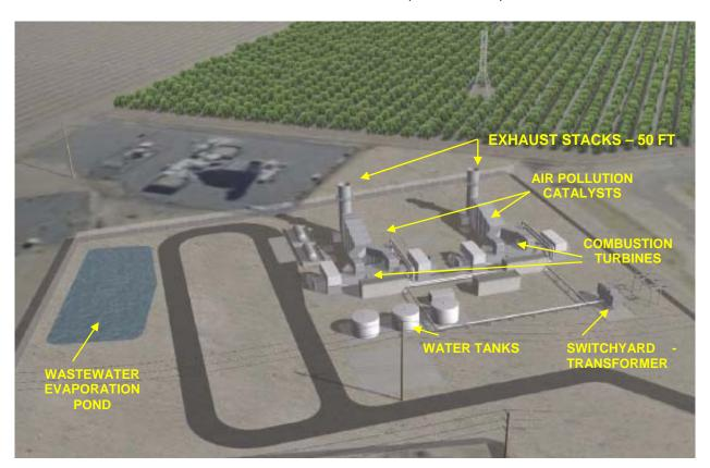
The SPP would not have a wet cooling tower; therefore, there would be no publicly visible water vapor plumes emissions. There is no potential for visible water vapor plumes to form from its exhaust stacks. The project would result in no visual effect related to publicly visible water vapor plumes. (FSA 4.12-11)
