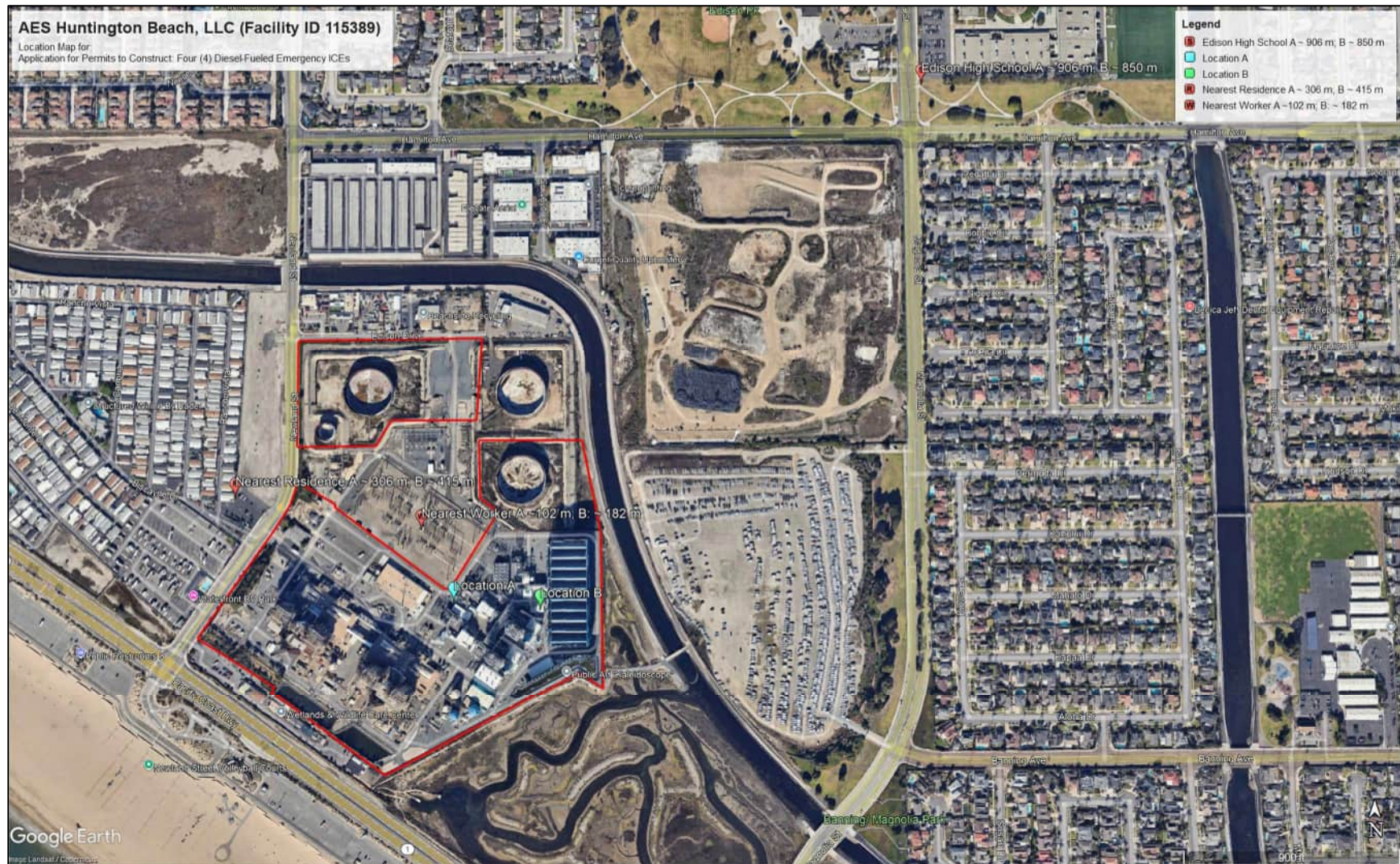
Figure 1-1: Aerial View of Locations A and B, and Surrounding Area
