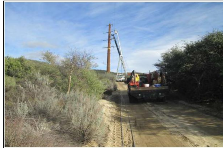
Typical power line (50-200 kV)
